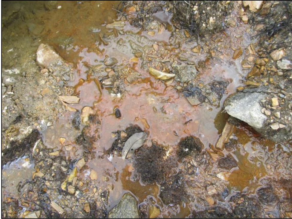
Figure 4. Site 1, showing iron hydroxide precipitate
