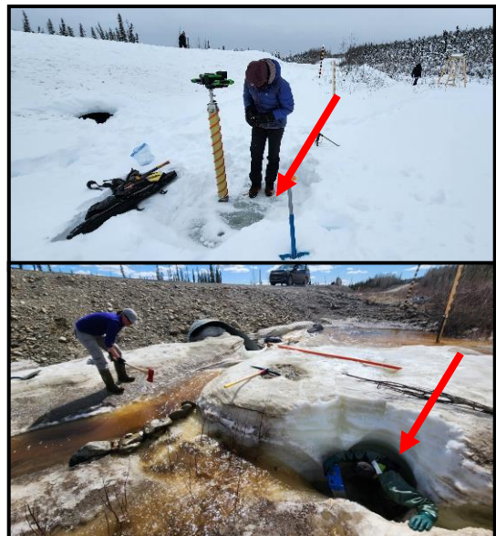
Figure 4. location of an augered hole at km 32.6 on the Dempster highway in March 2023 (top) and the expansion of this drainage hole by early May 2023 (bottom).
