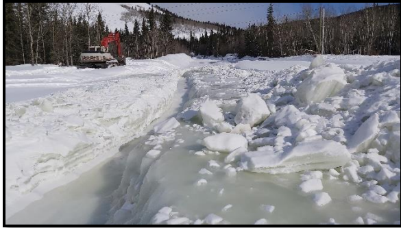
Figure 50. Ice excavation in March 2021 upstream of Jensen Creek culvert.
