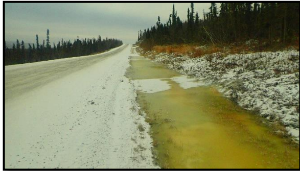
Figure 6. Groundwater-induced icing near km 29 on October 28, 2022.
