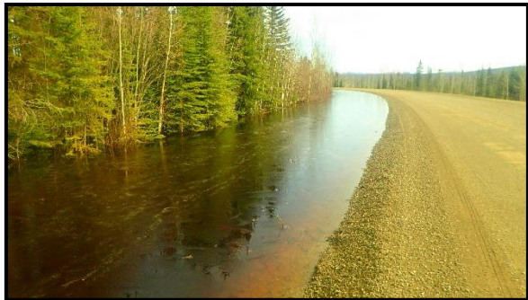
Figure 7. Water ponding on the upslope of the Dempster Highway near km 29 on May 9, 2023.
