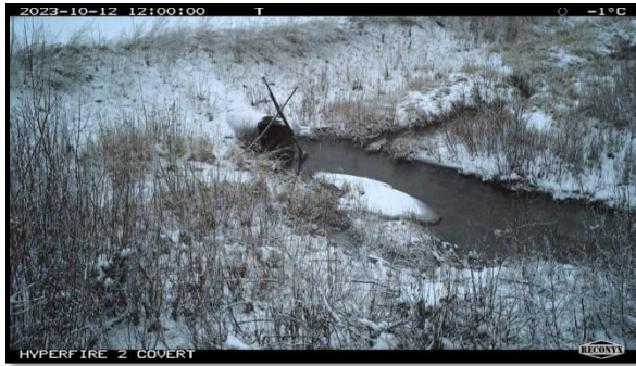
Figure 34. Timelapse camera photo of Unnamed Creek culvert head on Oct 12, 2023.
