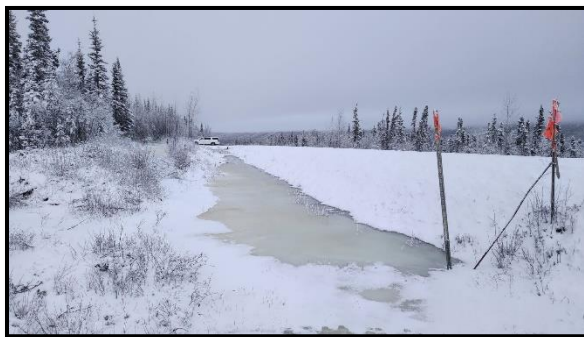
Figure 11. Unnamed Creek (km 33.8) culvert head and ditch on Dec 9, 2022.
