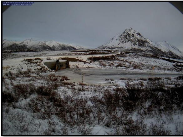
Figure 17. Timelapse photo of East Blackstone River culvert head on Oct 29, 2023.
