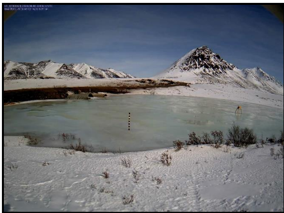
Figure 18. Timelapse photo of East Blackstone River culvert head on Apr 18, 2024.
