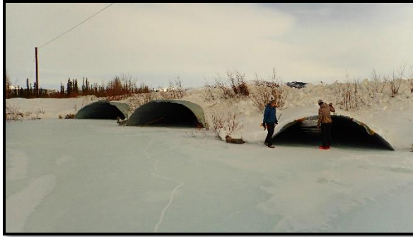
Figure 23. Engineer Creek at km 160.6 on April 3, 2024.
