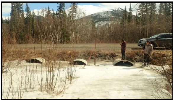
Figure 13. Yin Tang Creek culvert heads on May 8, 2022.
