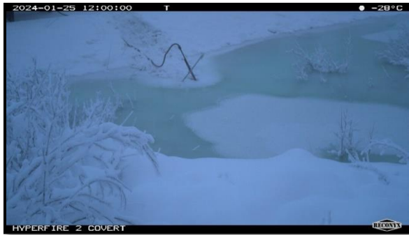
Figure 35. Timelapse camera photo of Unnamed Creek culvert head on Jan 25, 2024.
