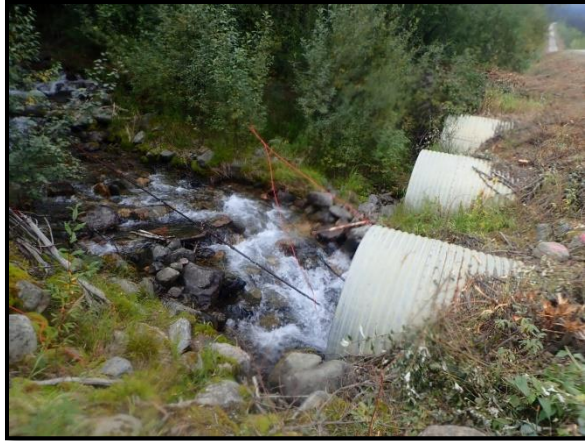
Figure 12. Yin Yang Creek (km 44) culvert heads on August 23, 2022.
