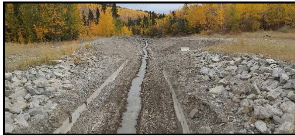
Figure 51. Newly excavated Jensen Creek channel upstream of culvert on Sept 18, 2023.
