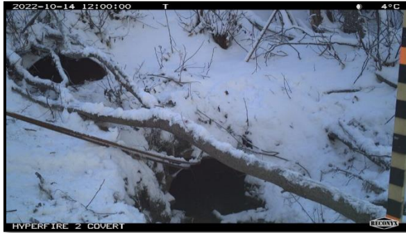
Figure 30. Timelapse camera photo of Lightning Creek culvert heads on Oct 14, 2022.
